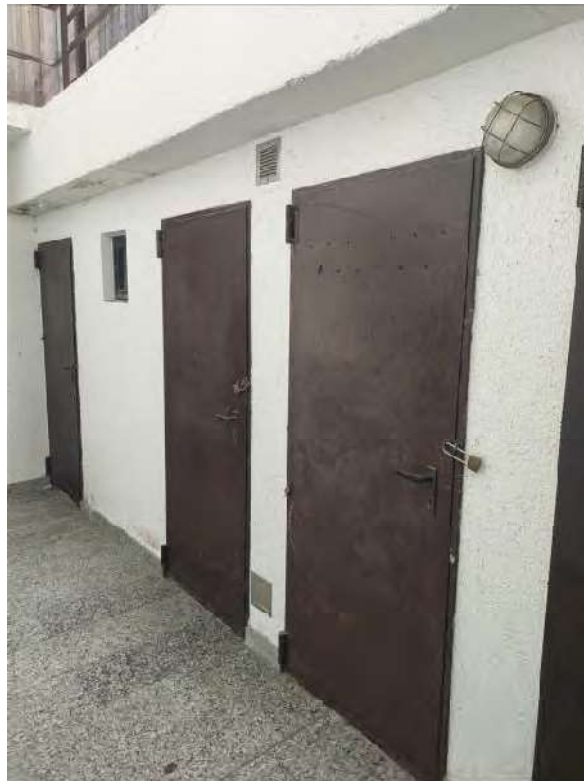
Cantine piano interrato
