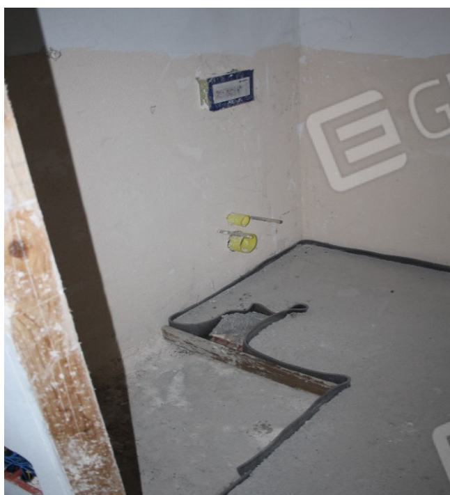
bagno piano terra
