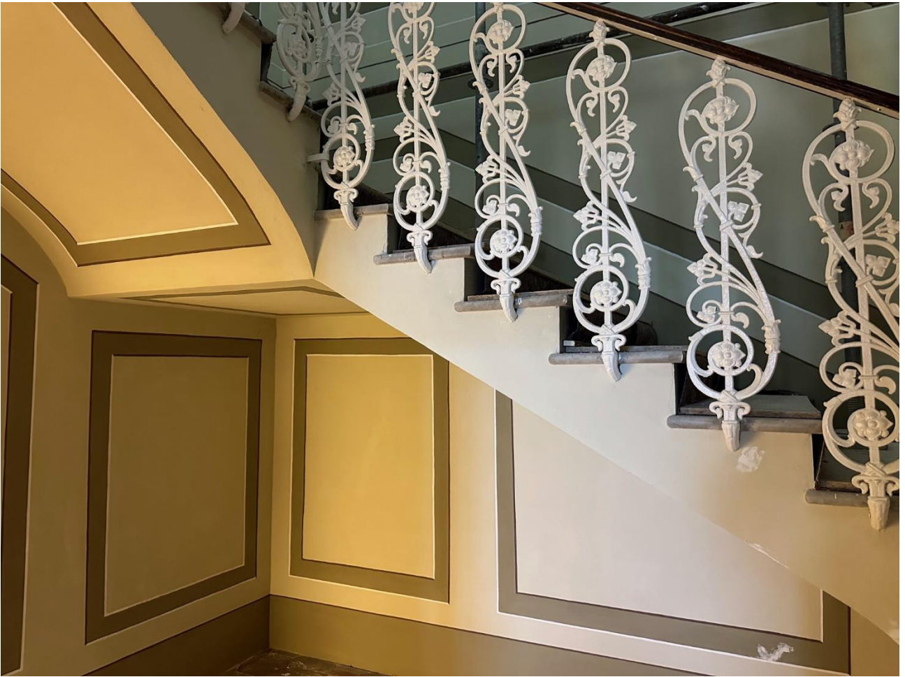
Scalone – Piano Terra
