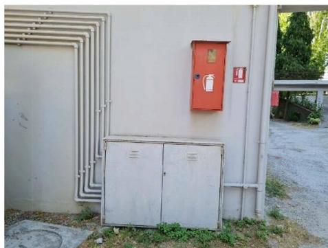
**FOTO 32** - CONTATORI GAS PER LA COTTURA DEI CIBI
